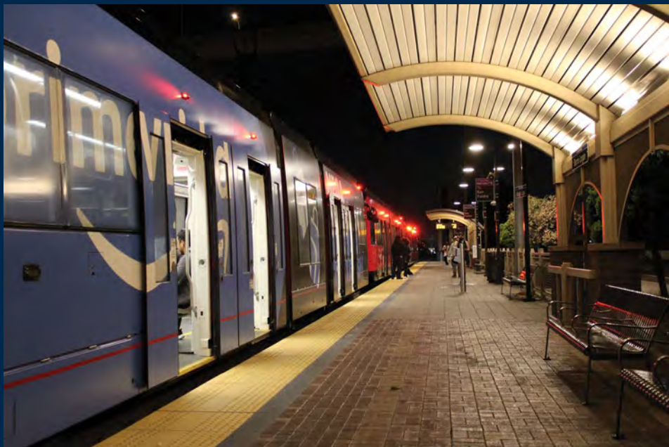
| San Diego Blue Line Station's Train Shelter Morrow Meadows Construction San Diego CA
